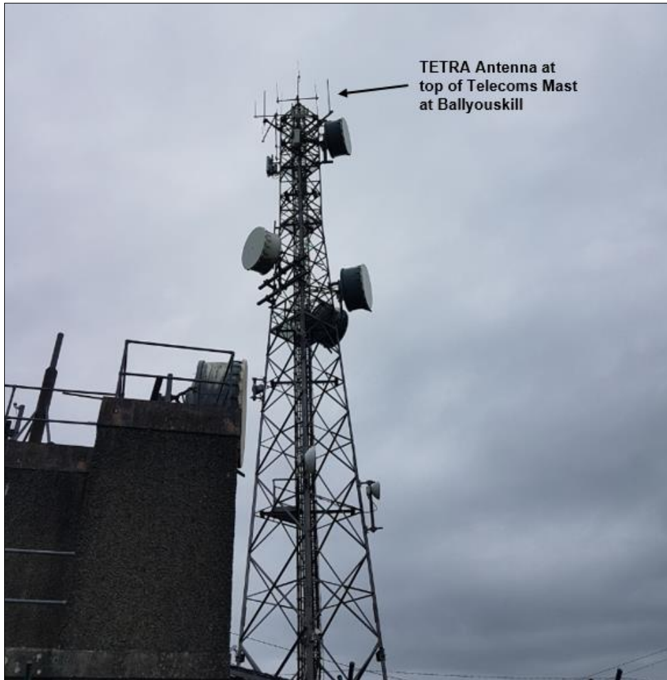
Figure 6. TETRA Basestation (LAC 4401) at Ballyouskill Mast-Site
